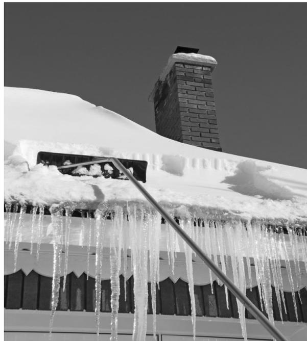
Snow rakes resemble a garden hoe with a long handle. Workers should be instructed to remove small amounts at a time to avoid strain or from being hit or buried by falling snow.
