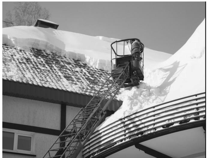
An aerial lift is being used in a snow removal operation. The worker is using a restraining belt and lanyard for protection.
