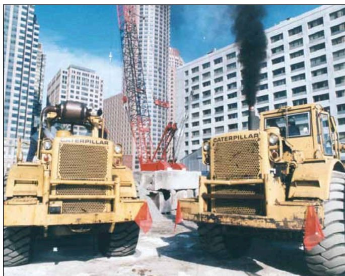
Heavy equipment operators can be exposed to diesel exhaust at construction sites.
